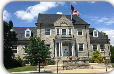
Borough of Carlisle Town Hall and Administrative Offices
